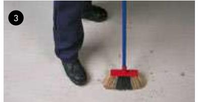
3- Surfaces to be tiled must be completely free of dust or any other substance which could impair tile adhesion. For specific installations (radiant heating systems, façades with mechanical anchors, ceramics on roofs/ceilings or particular design constraints) request additional information specifically for each application.
