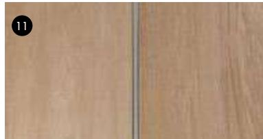
11- Take account of structural joints. Movement joints should be positioned as directed by the project designer. In general, do not design areas greater than 50-70 m<sup>2</sup> for interiors and half that for exteriors. Minimum joint width: 8 mm.
