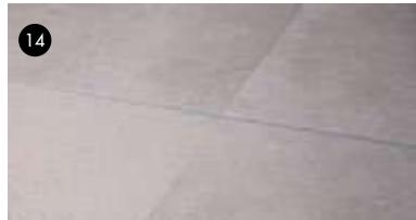
14- Joints should be grouted when the tiles are completely fixed to the substrate. In respect of paving, follow the recommendations of the adhesive manufacturer to ensure sufficient time is allowed before the floor is walked on or subjected to load. In this way movement and/or breakages are avoided.
