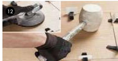
12- Both during installation and at the end of the day, check the quality of the work carried out before the bonding material sets. Correct any defects using suction cups and rubber mallets.
