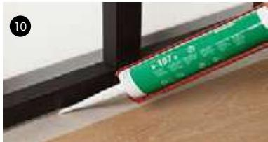
10- Edge joints occurring at corners, changes of paving level and changes of material should be covered with tile trim or a tile itself and sealed with flexible sealant. Minimum joint width: 8 mm.
