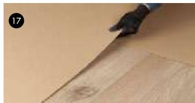
17- Protect the paving against premature loading, other construction work and adverse weather. We recommend covering the paving with sheets or boards to avoid a build-up of dirt and to protect from scratches, abrasion and impact.
