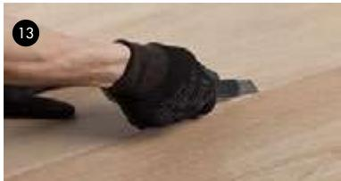
13- Prior to grouting, check that the bonding material has hardened. Remove the tile spacers, clean the joints along their length, width and depth, and check the joint is not damp.
