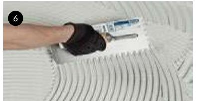
6- The only fixing system recommended is installation on a thin layer using a toothed trowel. A double bonding technique (with adhesive applied to both the substrate and the back of the ceramic tile) is recommended for tiles with a format larger than 1,000 cm<sup>2</sup> (33x33 cm).
