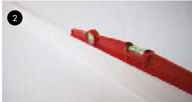
2- Check that the substrate to be covered is stable and the base is suitable for installing ceramic tiles: rough texture, not friable, completely flat and level. We recommend that all damp areas are waterproofed.
