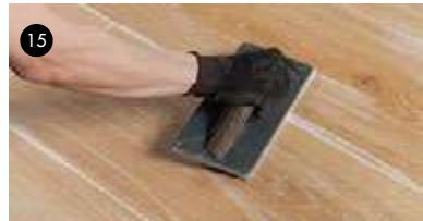
15- Follow the manufacturer's recommendations in respect of the preparation and use of grouting materials. Ensure that the material and tools chosen do not damage the tile surface. The grout should be applied using a rubber trowel. VENIS catalogues contain details of the butech materials recommended for each design.
